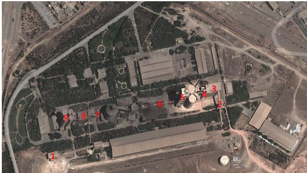
Figure 2: Perspective view of Tehran cement plant with tagged SPL measuring areas
